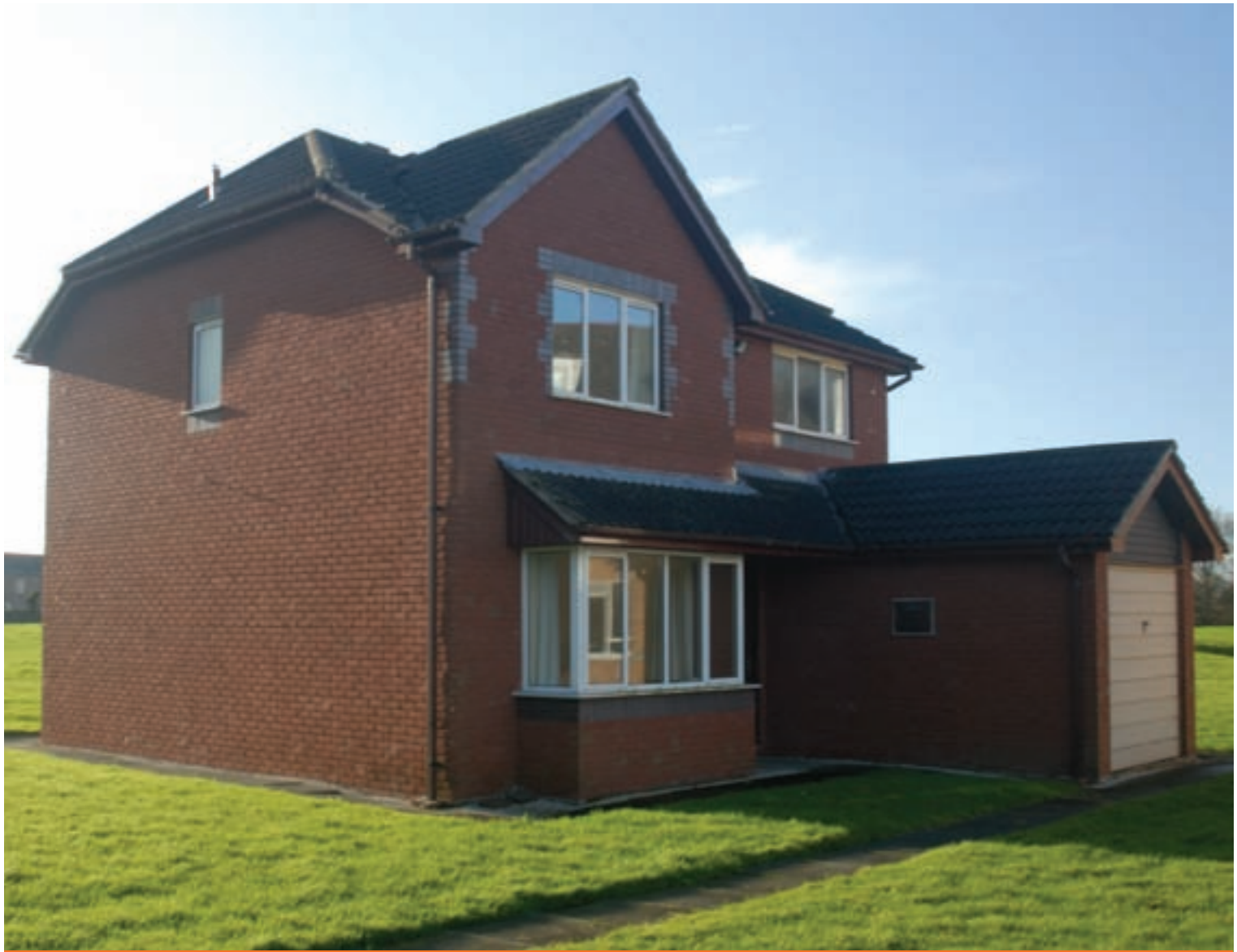
Above: Genlec field trial test house.
