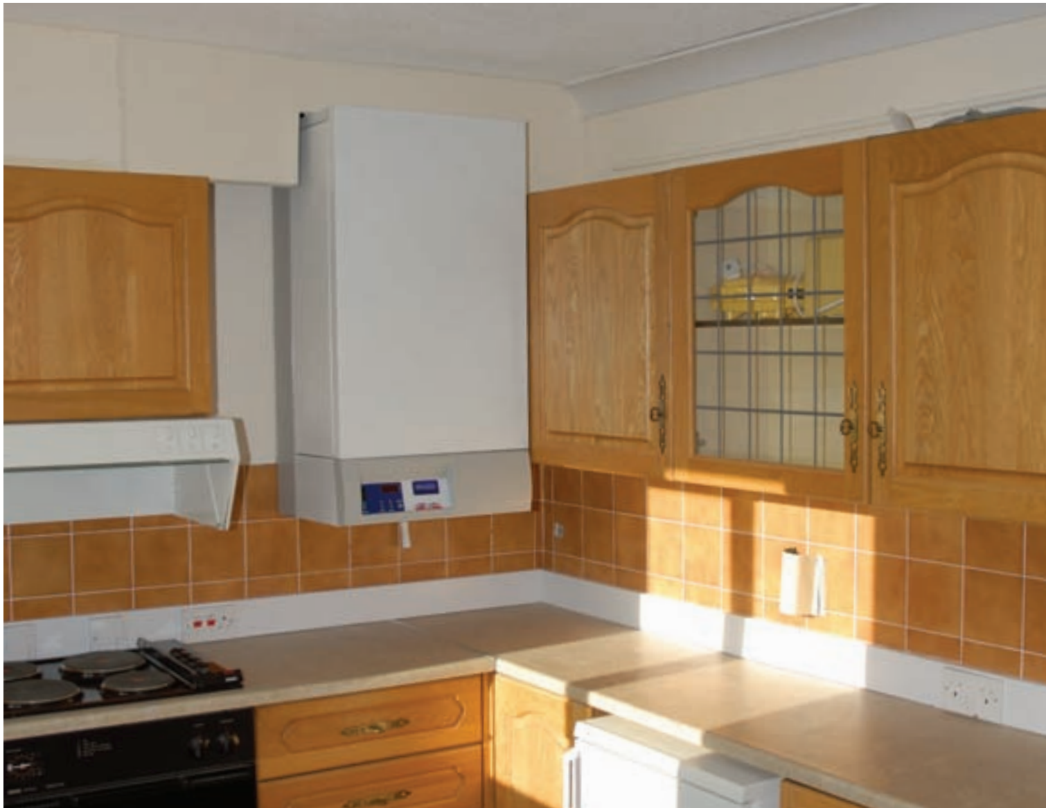
Above: Genlec's field trial mCHP boiler.
